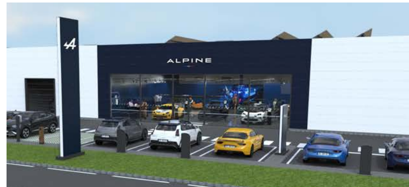
A complete identification of the Alpine facade
